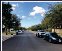
Crestwind Drive Between: Windrock Drive - Cul-de-sac
