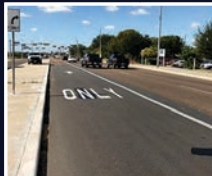
Del Mar Boulevard Windfield Parkway Turning Lane Extension
